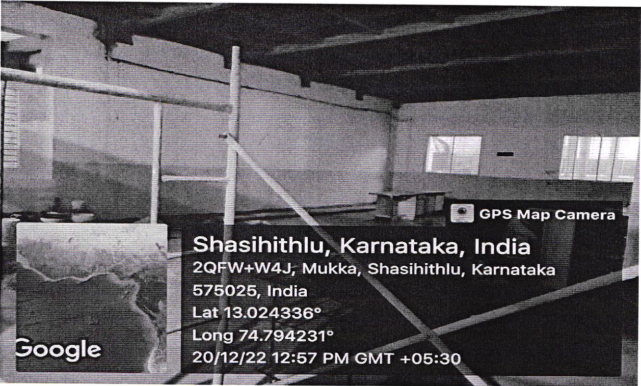
CLASSROOM 93 (under renovation)
